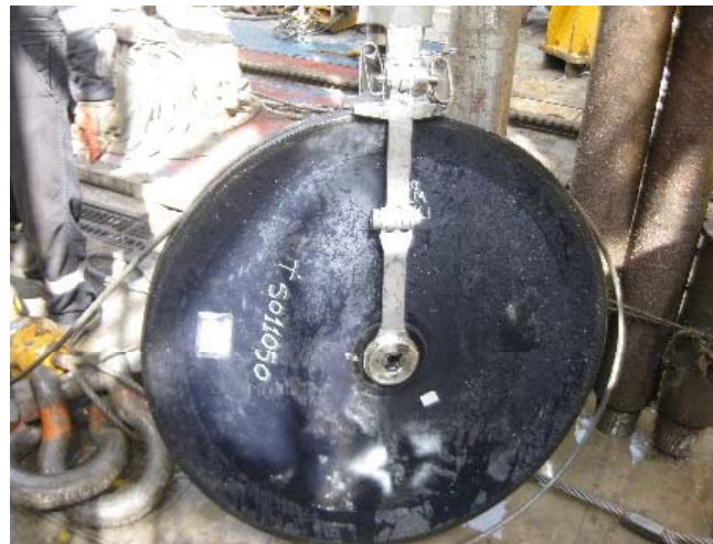
Unguarded crown Sheave
